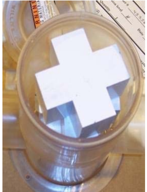
Chlorine correctly installed
